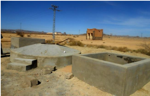
Fig. 9 Biogas digester with a capacity of 15m 3 installed at Tamanrasset city (Southern of Algeria).
